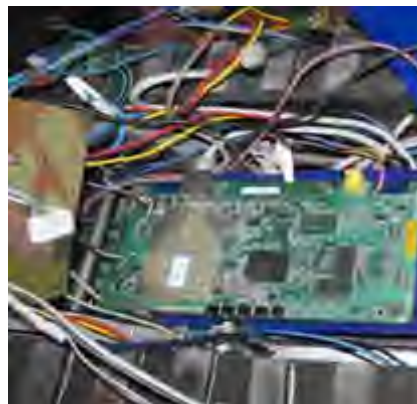
Fig. 3. Dlink Access Point Board
